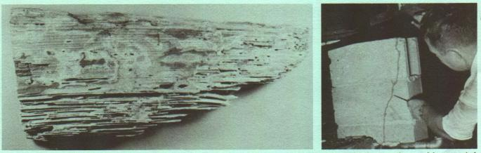
Fig. 12. (Left) Douglas fir plank damaged by termites. Note remaining harder summerwood and debris on surface and in excavated parts of wood. Fig. 13. (Right) Termite shelter tubes built over concrete block support under wood framed structure.
