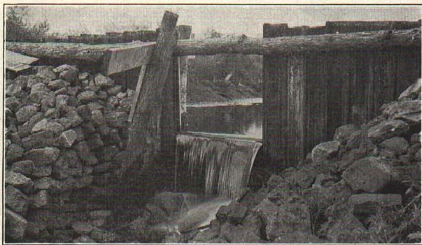
Figure 7.—The most successful grower is the one who has the water supply in his muck at his control. This picture shows one of the most efficient types of dams, constructed of interlocking sheet steel piling driven well into the muck and reinforced by rock piled on the lower side.
