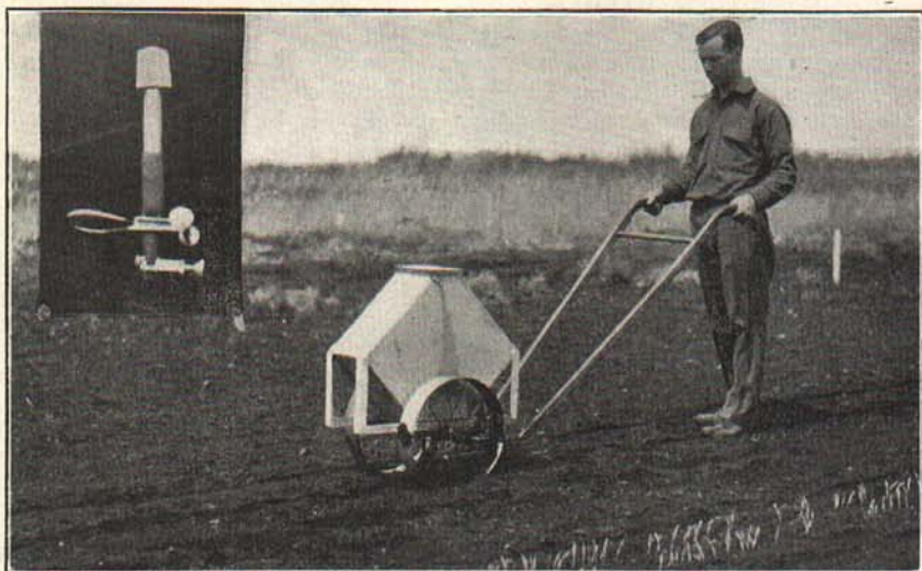
Figure 13.—A home-made distributor for corrosive sublimate treatment for maggot control. The tank attaches to a wheel-hoe frame and is of galvanized sheet iron reinforced with angle iron, the inner surface of the tank being covered with asphaltum paint. Dimensions of tank 20 x 20 x 8 inches, with one edge removed to give an 8 x 8 inch base, and the opposite edge removed to give a 6 x 8 inch opening in top. Capacity of tank 12 gallons, sufficiently large for treatment of a row 50 to 60 rods long. The distributing pipe ends in a piece of rubber tubing on which is attached a screw clamp by which the flow is regulated. A pinch clamp is used to close the rubber tubing when flow is not desired. The distributing pipe must be in line with the axles of the wheels and the lower end in plain view of the operator so that the flow can be directed on the onion row. Inset shows distributing pipe with rubber tubing and clamps attached. Three-inch sheet iron rims on wheels facilitate the handling of the machine while a cheese-cloth strainer prevents clogging of the distributing tube.
