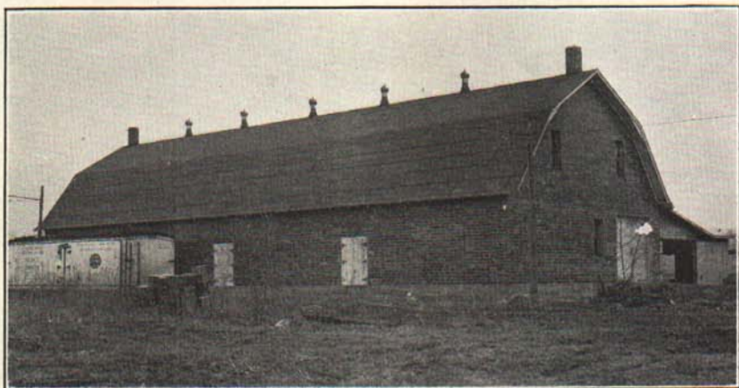
Figure 16.—A 60-car storage constructed of glazed block tile. Built on a siding, the onions are loaded directly from the storage into the car. On the farther side the covered driveway offers protection for loads in inclement weather, as well as storage for empty crates.
