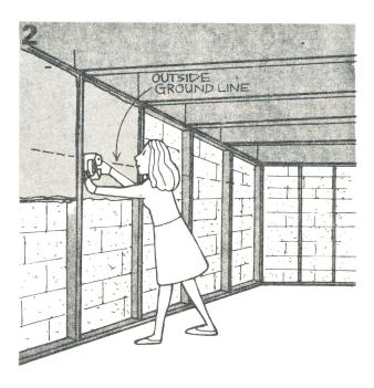
Cut blankets into sections long enough to extend from the top plate to 2 feet below the ground line. Staple them into place between the studs, with the vapor barrier towards the living space. **NOTE**: in northern climates there will be added benefit to installing the insulation the full height of the wall.
