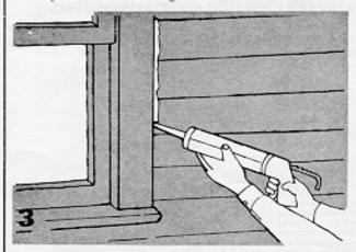
A wide bead may be necessary to make sure caulk adheres to both sides.
