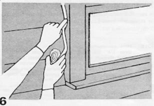
Caulking compound also comes in rope form. Unwind it and force it into cracks with your fingers. You can fill extra long cracks easily this way.
