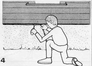
Fill extra wide cracks like those at the sills (where the house meets the foundation) with oakum, glass fiber insulation strips, etc.)
