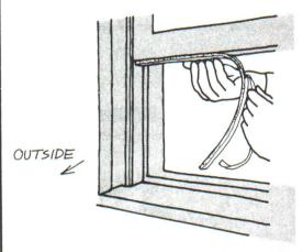
Install adhesive backed foam, on all types of windows, only where there is no friction. On double-hung windows, this is only on the bottom (as shown) and top rails. Other types of windows can use foam strips in many more places.
