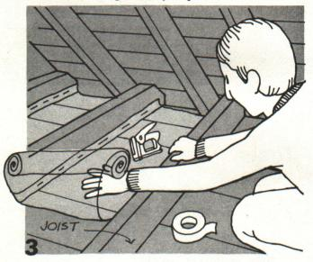
Install separate vapor barrier if needed (see page 4). Lay in polyethylene strips between joists or trusses. Staple or tack in place. Seal seams and holes with tape. (Seams may be overlapped 6" instead.)
