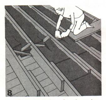
Cut ends of batts or blankets to fit snugly around cross bracing. Cut the next batt in a similar way to allow the ends to butt tightly together. If page 42 calls for an **R-Value** that requires a second layer, place it **at right angles** to the joists.
