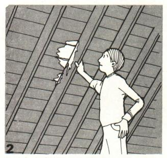
Check for roof leaks, looking for water stains or marks. If you find leakage, make repairs before you insulate. Wet insulation is ineffective and can damage the structure of your home.
