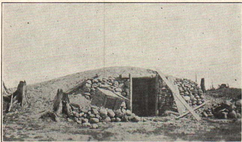
Fig. 2.—An excellent use of field stone. Such a house is economical, easily constructed and durable.
