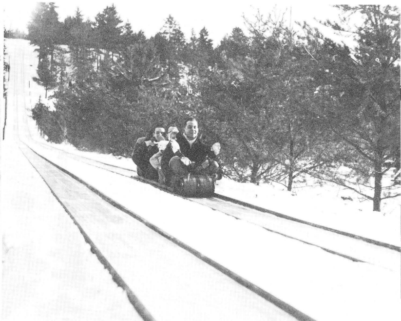
Fig. 8. Typical toboggan run with steel rail sides. Note straight route and absence of dips or bumps. Proper construction and layout are needed for safety.
