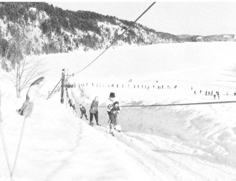
Fig. 9. Rope tows are very popular because of capacity, ease of installation and low cost. Proper installation reduces rope breakage.
