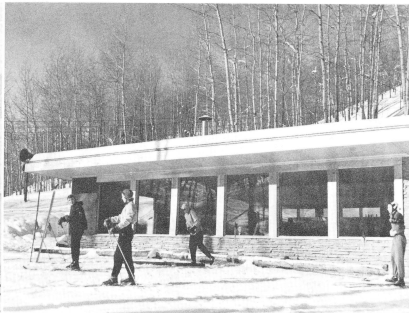
Fig. 17. All buildings should be attractive as well as functional, easily maintained, suitably sited, and easily expanded in future.
