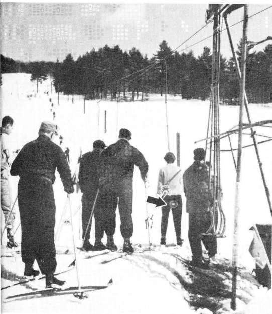
Fig. 11. Platter Pull. A durable type; takes up one skier at a time. Capacity can be adjusted to need.
