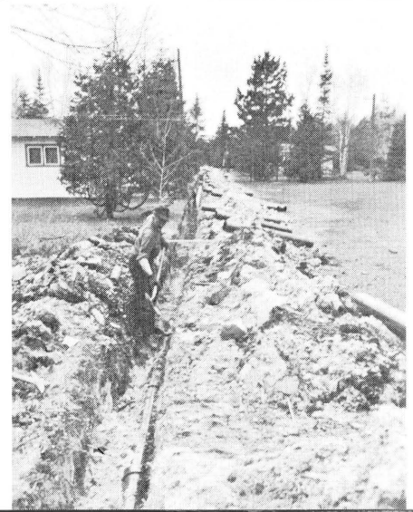
LAYING SEWER TILE
