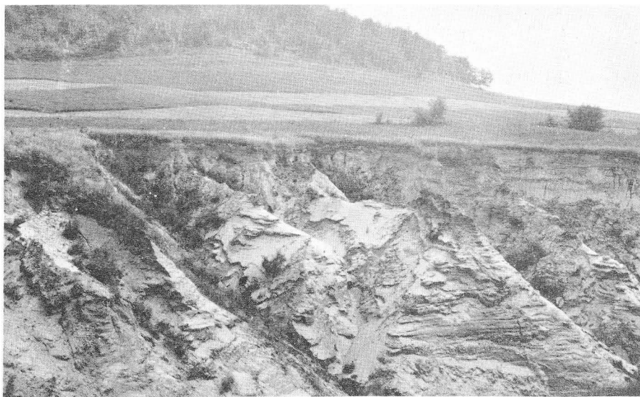
Fig. 4. Gully in Buffalo County, Wisconsin, showing deep bed of river terrace sand (U. S. Forest Service).
