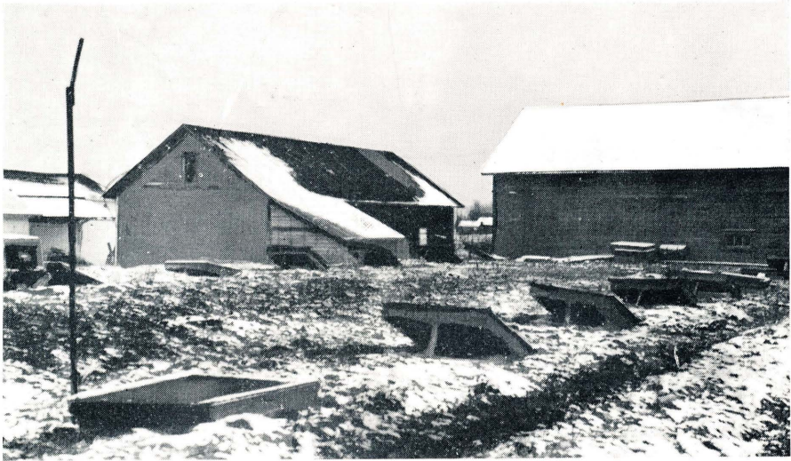
Fig. 8. Ceiling hatches of storage cellar. Potatoes are often injured in filling storages through such hatches even when sack or padded chutes are used. The accumulation of a cone of dirt under the hatches is also undesirable.
