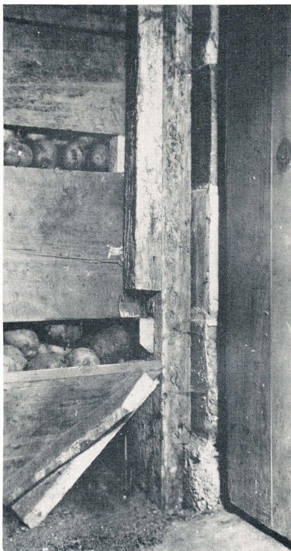
Fig. 11. Interior view of the Lake City storage showing entrance of triangular wall-floor air flue which connects the open work alley with a two-inch wall air circulation space. Later practice uses tight bin fronts.
