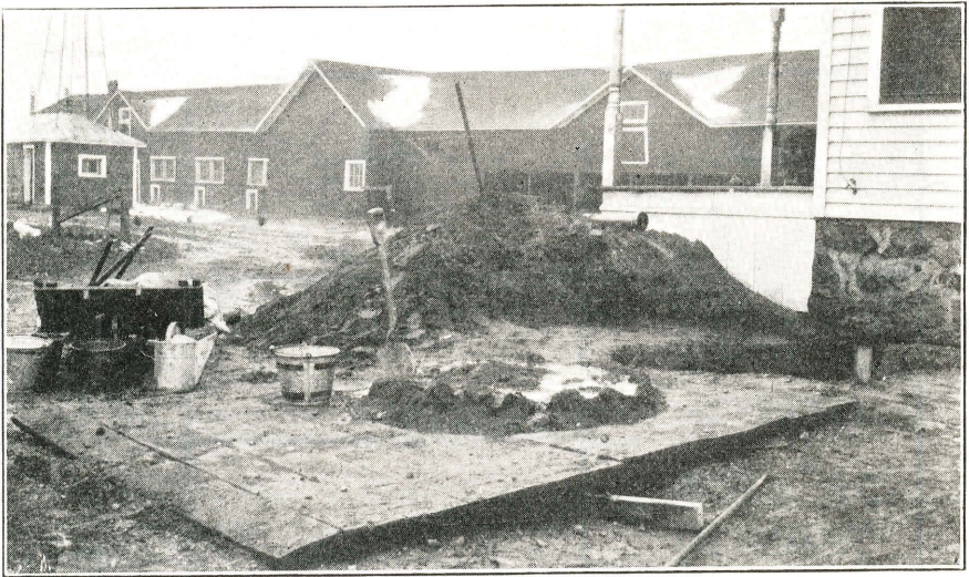
Fig. 7.—If a mixer is not available concrete may be mixed to best advantage on a platform.
