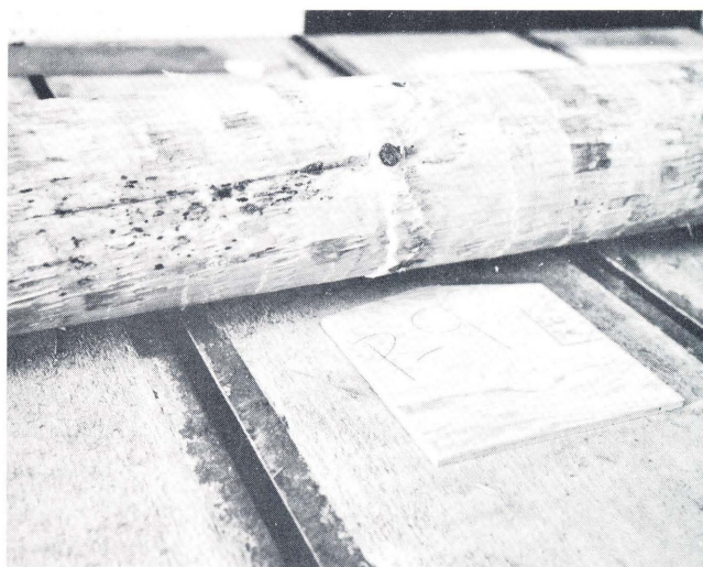
Fig. 11. Compression failure in pole P-9.
