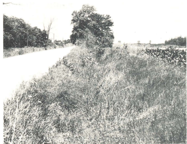
Fig. 15. Ditches plugged with brush and trash retard the rate of water removal. This situation increases opportunities for soil compaction and crust formation.
