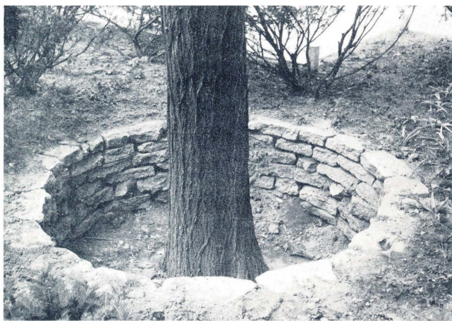
Fig. 4. Stone, cement blocks, and other material may be used to build a tree well.
