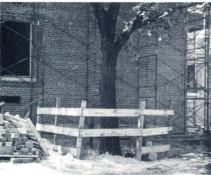
Fig. 1. Boxed-crate structure 10 feet square around a tree.
