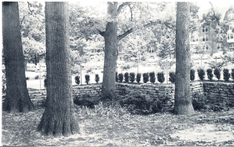
Fig. 5. This retainer wall protects several trees from fill.
