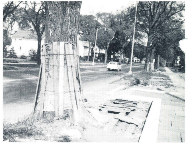
Fig. 2. Slats woven around a tree trunk to prevent scarring of the bark.
