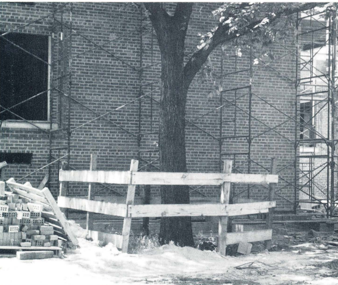
Fig. 1. Boxed-crate structure 10 feet square around a tree.
