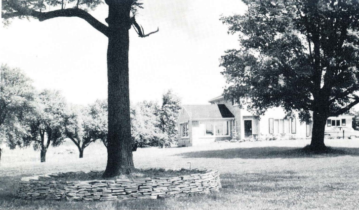
Fig. 6. A retaining sandstone wall protects roots from excavation.
