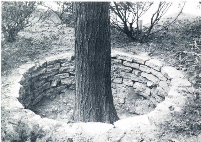
4. Stone, cement blocks, and other material may be used to build a tree well.
