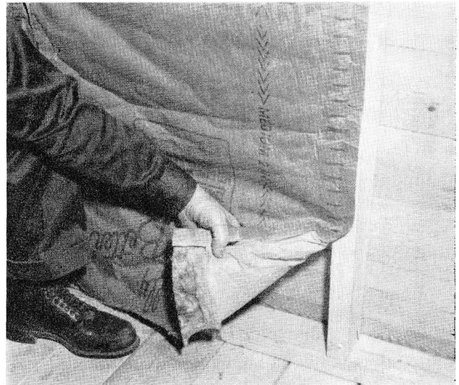
Figure 3. Providing a nailing flange at the bottom of blanket insulation for nailing to the sill.
