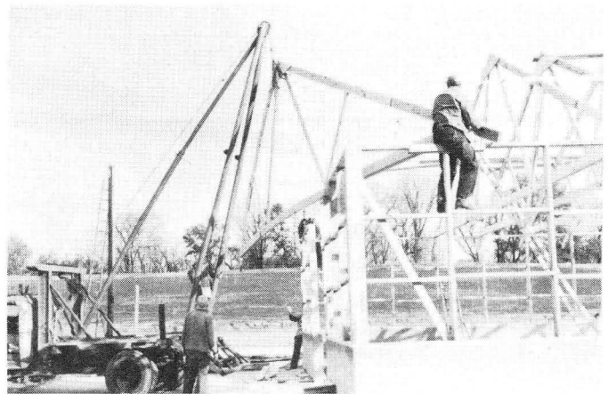
Fig. 18. Hoisting equipment may be needed to erect larger trusses on high sidewall buildings.
