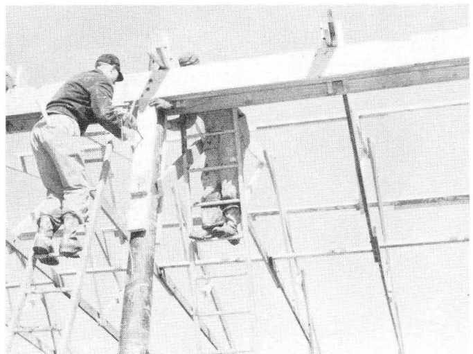
Fig. 19. The proper anchorage of the rafter supports, with scabs bolted in place, is important in pole frame buildings. All of the roof load is transferred to the sidewall poles in this case.
