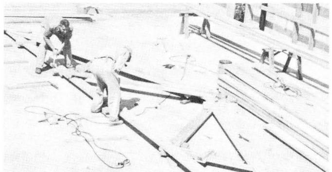
Fig. 6. For this trussed roof poultry house, the ring-bolt truss members are being drilled in a jig. The jig holds all members in the exact position they will have in the truss. Once the holes have all been drilled straight and accurately, the members are removed from the jig, grooved, and assembled into a truss.
