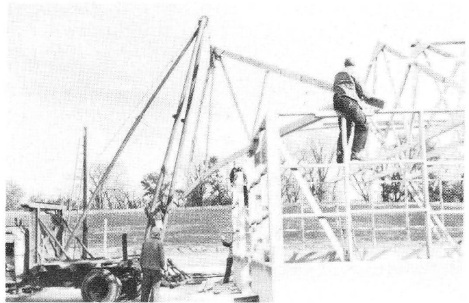
Fig. 18. Hoisting equipment may be needed to erect larger trusses on high sidewall buildings.
