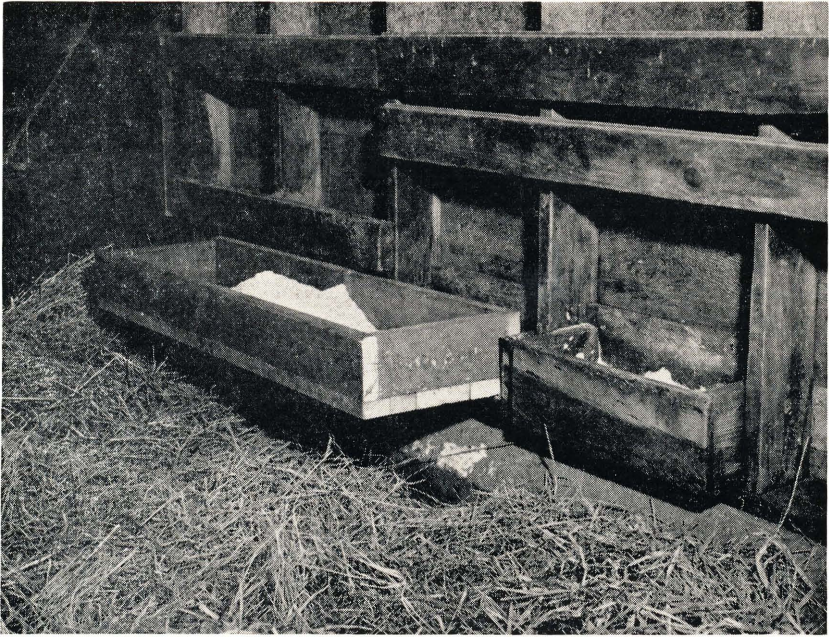
Fig. 18. Feed box for fattening steer. Notice that it is constructed of 2 x 6 inch planks and is spiked to the wall so that the steer feeds at a convenient height. Next to it is a box for salt—or a mixture of salt, steamed bone meal, and ground limestone.
