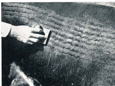
Fig. 3A. Using the "marking" or "lining" comb.
