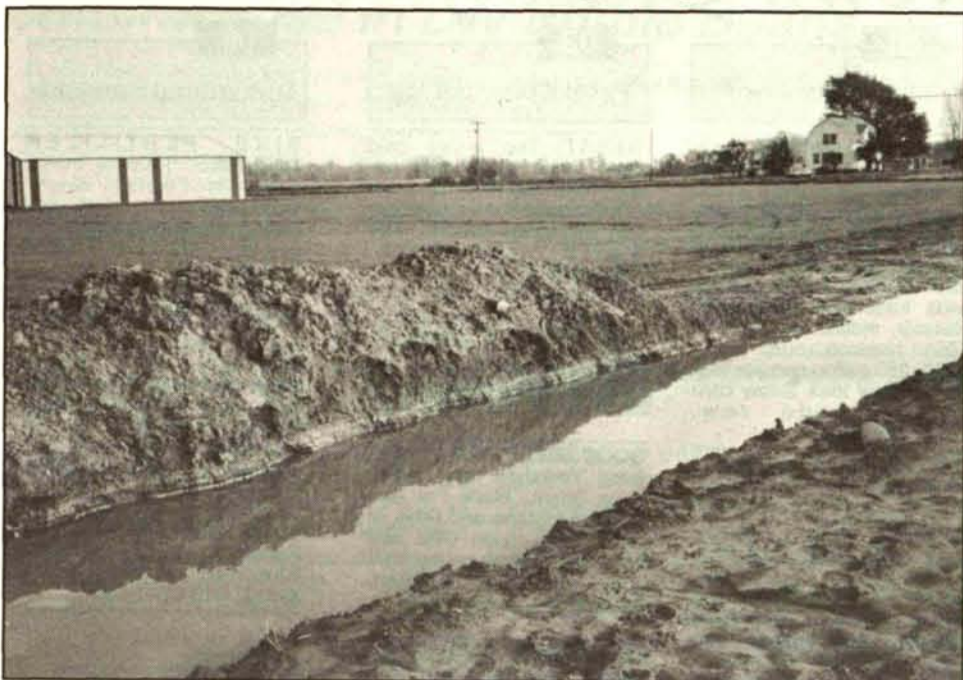
The 16 inch trench originally agreed to between the pipeline company and landowners grew into a ditch six to eight feet wide and 12 to 15 feet deep (at left) that was dug six weeks in advance of the pipeline laying crew (below). During that time, several heavy rains and cut field filled the ditch.
