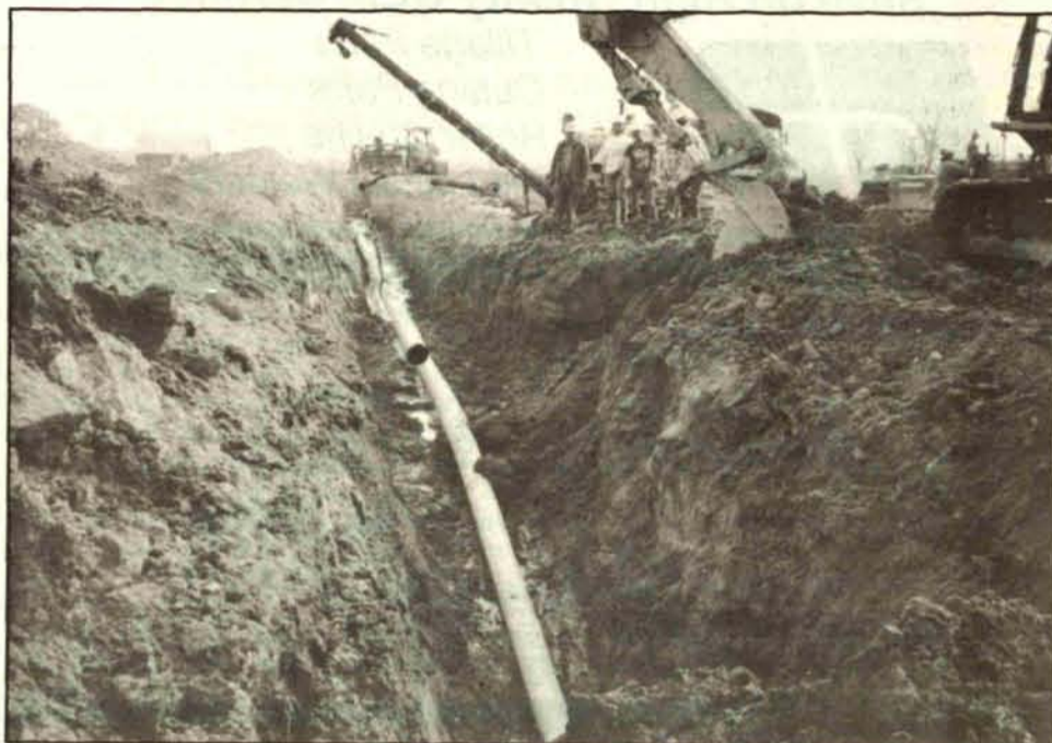
The 16 inch trench originally agreed to between the pipeline company and landowners grew into a ditch six to eight feet wide and 12 to 15 feet deep (at left) that was dug six weeks in advance of the pipeline laying crew (below). During that time, several heavy rains and cut field filled the ditch.
