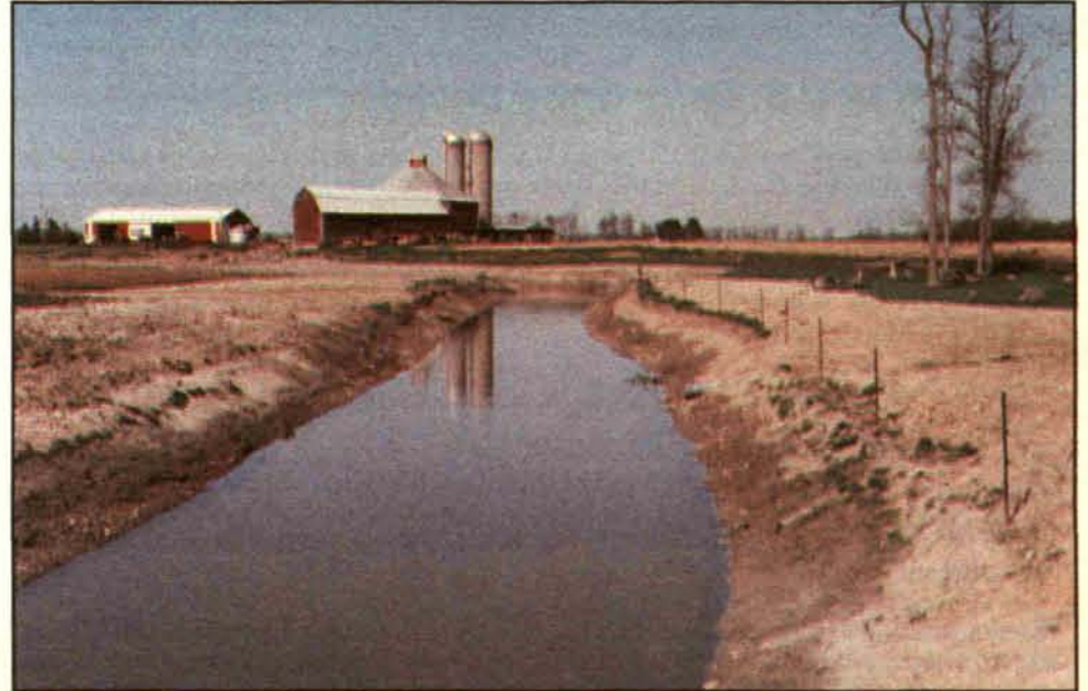
This portion of the drain is part of the seven-mile extension of the Philp drain that is at the heart of the controversy and threatens a $1.5 million project and a 4-year process to improve the drain.
