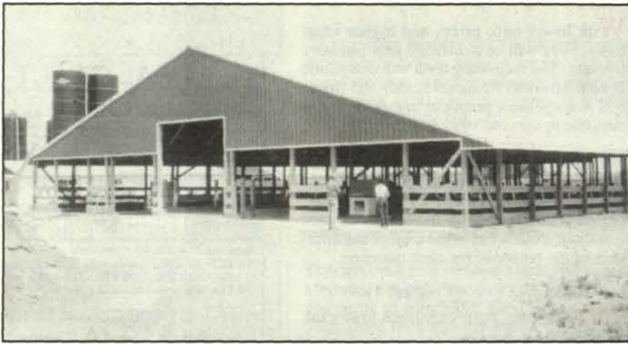
This 250 cow freestall barn, with curtain sidewalls, was put into operation on the Nobis dairy farm near St. Johns, in 1988. The ends of the barn also open and close.
