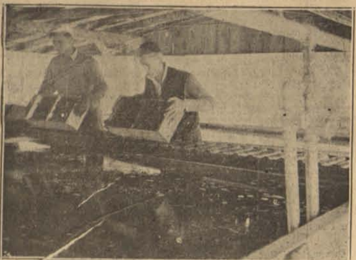
2 Second stop for cherries is the cooling and washing vat. Cold water hardens the fruit for the mechanical pitters. Each of nine tanks like this one holds 7 tons of cherries.
