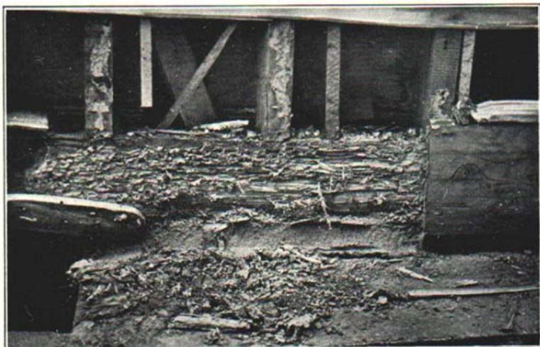
Fig. 5. Foundation destroyed by termites.
