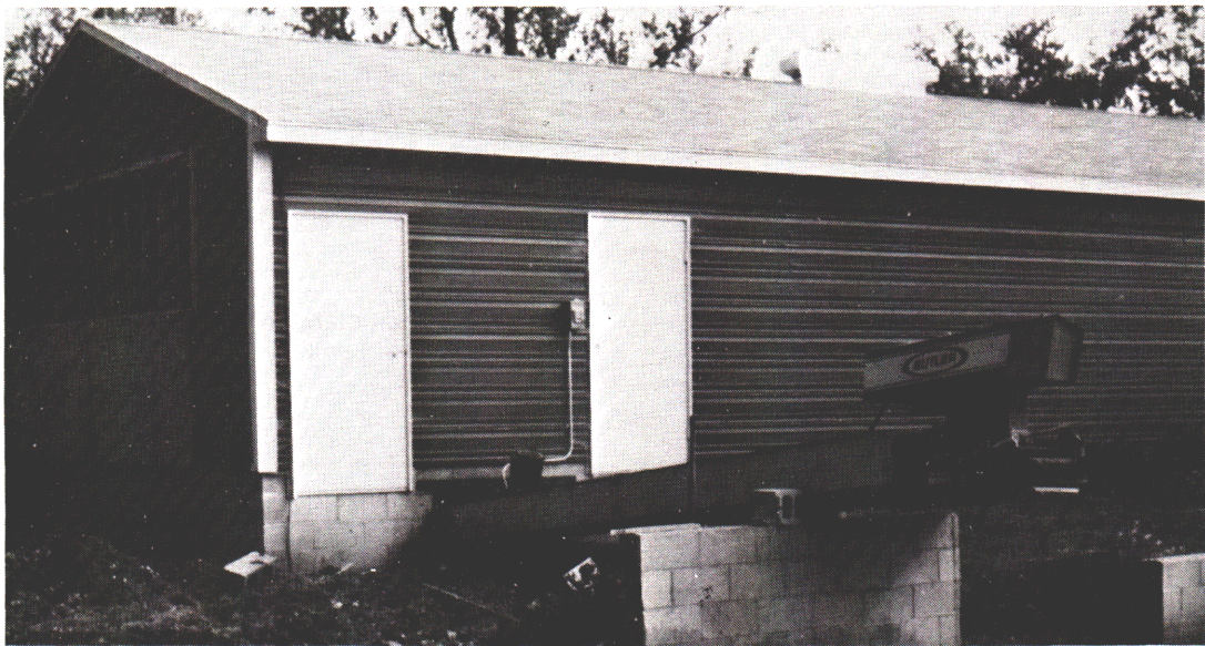
Figure 6. Traditional gutter cleaners work well in a solid manure system.
