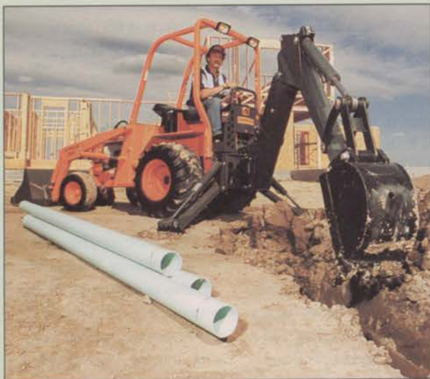
The Allmand Bros. tractor-loader-backhoe is rugged.
