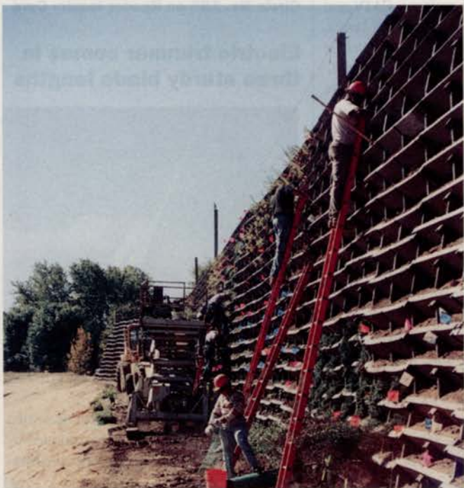
Kuehne Company built this 22-foot-high traffic noise barrier using triangular-shaped frames of recycled plastic called Recy-walls by Sanders Enterprises Inc.
