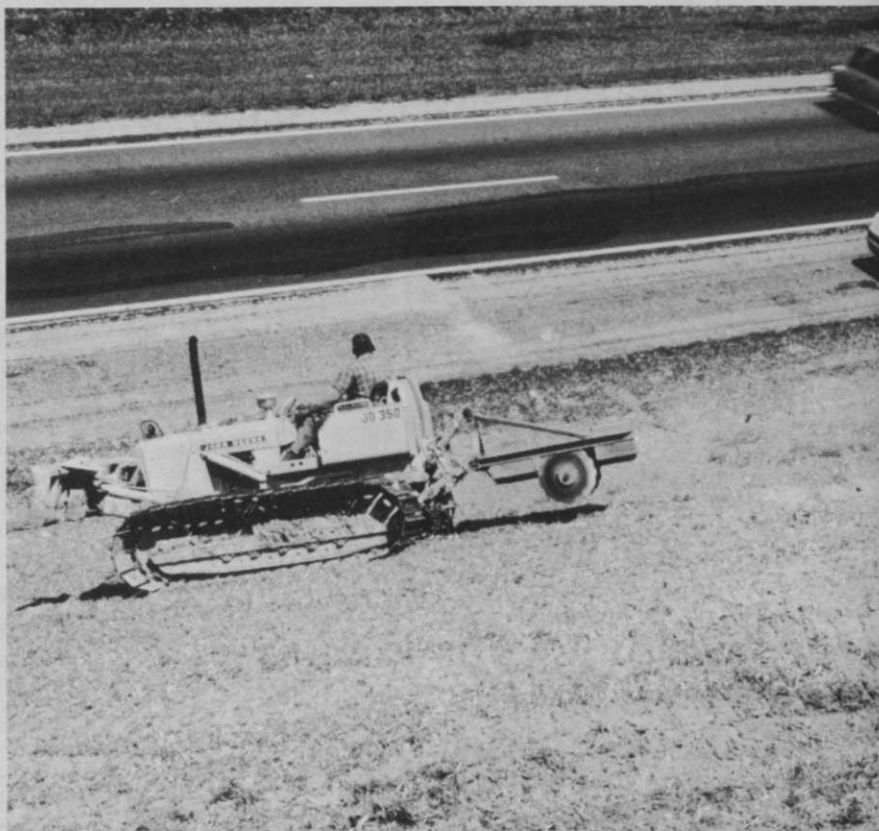
Mulch anchoring tool for incorporation of seed and mulch with soil requires heavy power unit. Work was done on the John F. Kennedy Memorial Highway in the state of Maryland. Effort was a government research project in cooperation with state.
