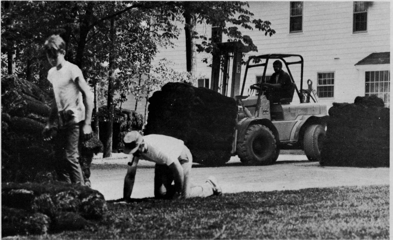
With the lift, Emerald Valley Sod is strategically stock-piled on the job site. Installers have learned this service cuts "travel time" by two-thirds on the average front home lawn.
