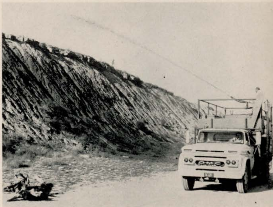
Conwed Hydro Mulch is being applied in this instance to a typical slope by hydraulic method. Seed, mulch and fertilizer are mixed, then applied on soil at distances up to 100 ft.
