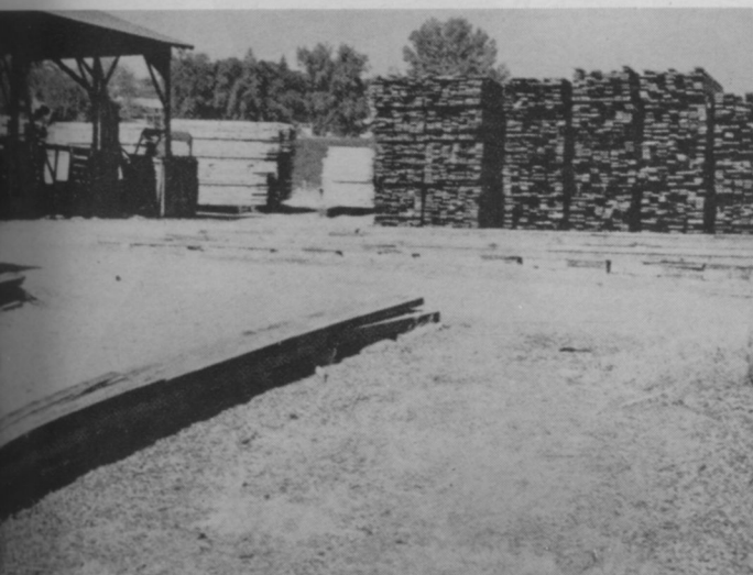
Fire-hazardous vegetation was controlled with Hyvar® X bromacil weed killer in the lumber yard area above. "Hyvar" X is a wettable powder formulation for use in sprayers equipped with adequate agitation. After application "Hyvar" X gives the same effective control as new "Hyvar" X-WS. All Du Pont weed killers are non-volatile, non-flammable, non-corrosive and low in toxicity to man and animals when used as directed.
