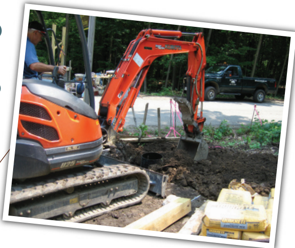
David DeFranco, president of DeFranco Landscaping, excavating with a Kubota U35.
