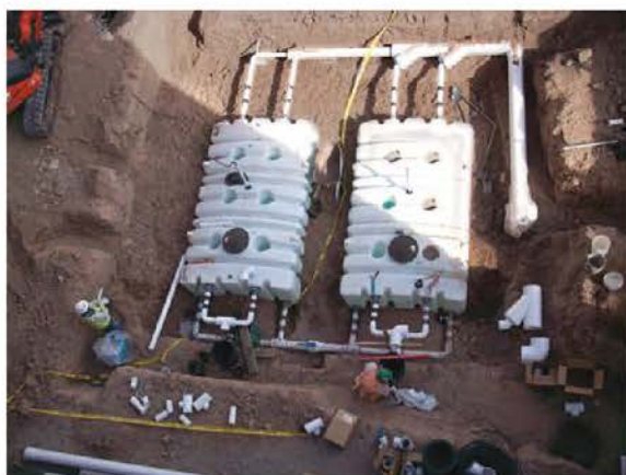
Heads Up Landscaping workers construct two rainwater harvesting tanks in the courtyard of the Silver Gardens Apartments in Albuquerque, NM (left). The finished photo (above) shows the same area after landscaping, from a slightly different perspective.
