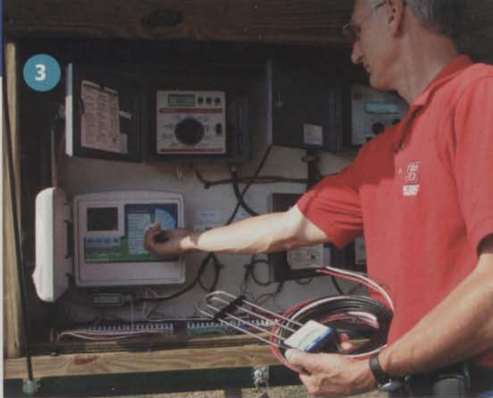
The project at the NCSU Lake Wheeler Turfgrass Field Lab seeks practical information concerning turfgrass irrigation. 1 Dr. Bir Thapa with soil-water moisture probe. 2 Back side of controller box with atmometer (left) and weather station (right). 3 Dr. Grabow at the controls of the "on-demand" system that NCSU is evaluating. 4 Grad student Arjun Vasanth installs a soil-water sensor.
