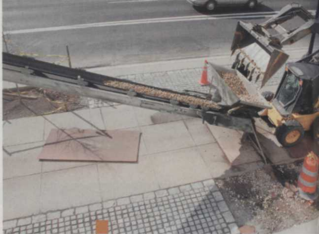
McDonnell Landscape lifted the green media to the roof with a Telebelt.
