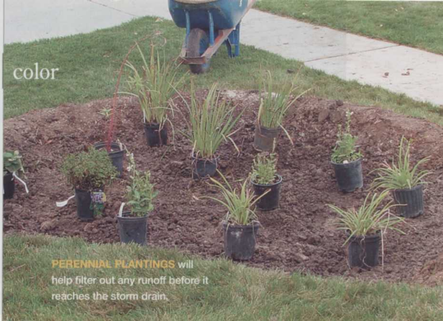
WHEN EXCAVATING a rain garden, be sure to leave a lip of soil on the downhill side of the newly dug swale.
