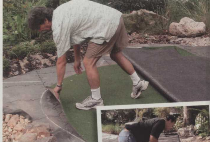
The interlocking panels cut installation time by as much as 70 percent and do not require any large equipment.
