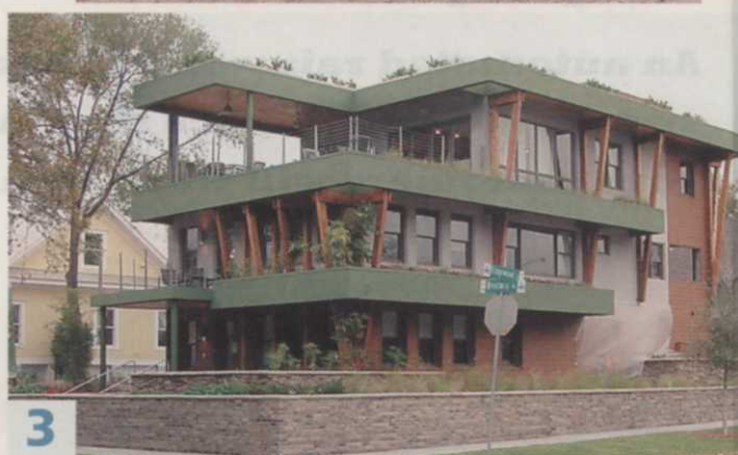
1. The design of the recovery-piping network is custom to each home and can include roof, patio and deck plantings and collection drains strategically placed around the home or facility property. 2. An underground cistern holds the water until it is needed for irrigation. 3. A customized rainwater recover system for this flat-roofed “green” home in Orlando helped it earn the New American Home 2007 award at last year’s National Association of Home Builder’s International Builders’ Show.
