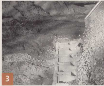
PHOTOS COURTESY : KEYSTONE RETAINING WALL SYSTEMS, INC.
