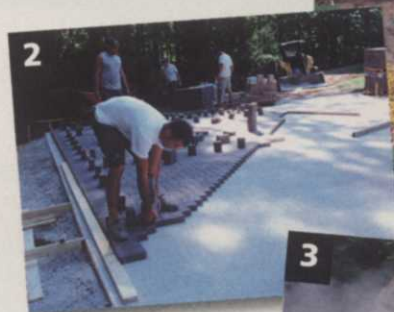
The Outside Design crew excavated (1), cut and laid pavers (2, 3) over a two-and-a-half week period to create the finished court.
