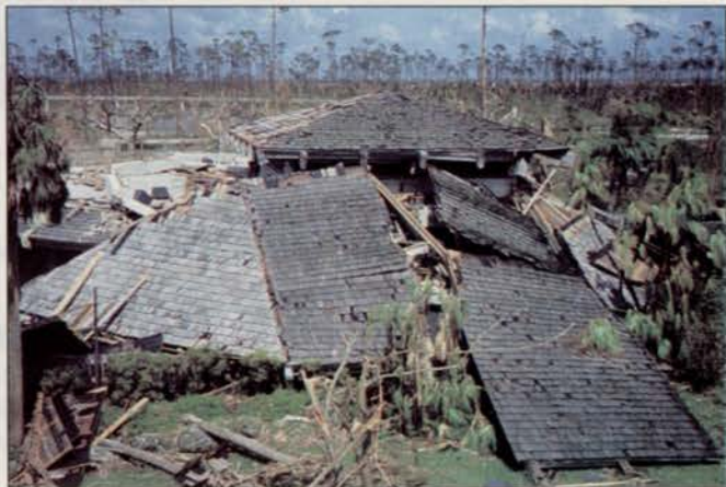
Hurricane Andrew destroyed the zoo's Lakeside Restaurant.
