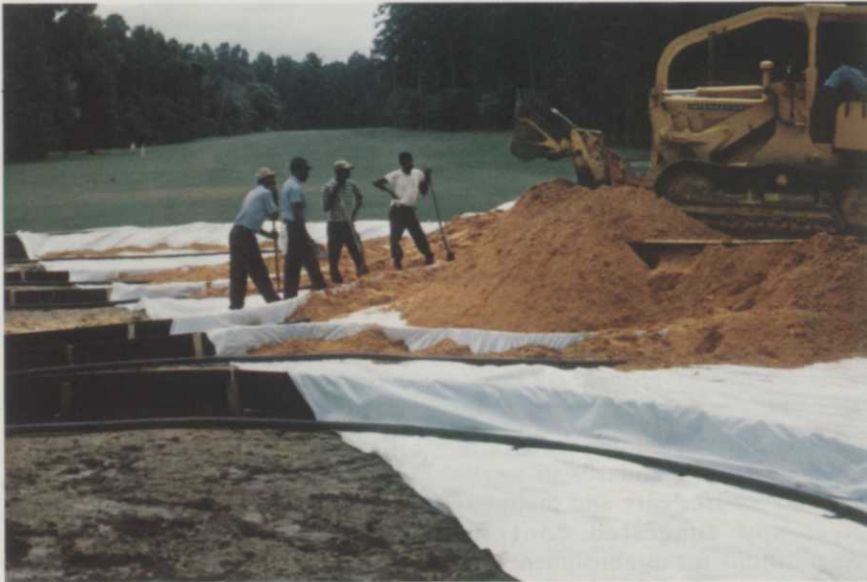
Spreading Sand over Tu-Tuf barrier on model green, 6 compartments, showing drainage pipes in each compartment.
