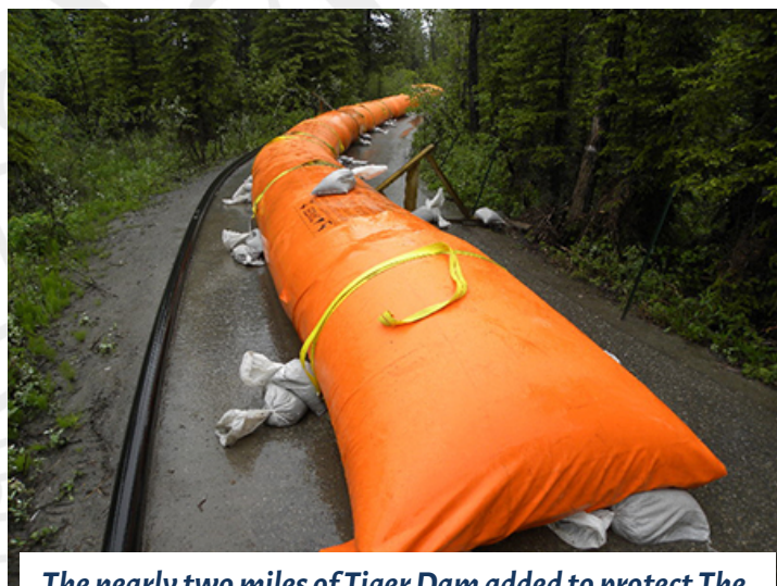
The nearly two miles of Tiger Dam added to protect The Glencoe Golf & Country Club was definitely good insurance. Note: the white mark on the tree to the right which shows the height of the river the year before.
