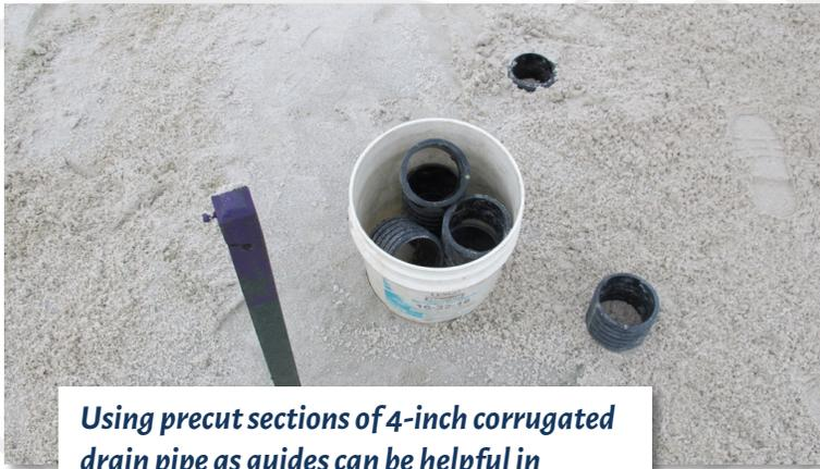
*Using precut sections of 4-inch corrugated drain pipe as guides can be helpful in maintaining proper sand depth in bunkers.*
