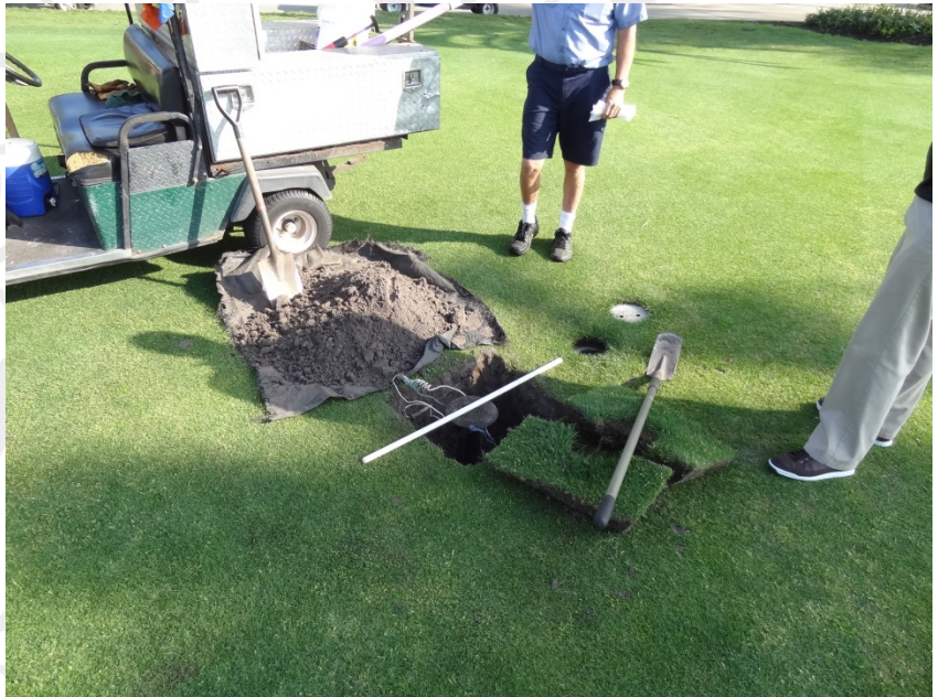
Figure 1 - Raising and leveling irrigation heads helps improve distribution uniformity and water-use efficiency.
