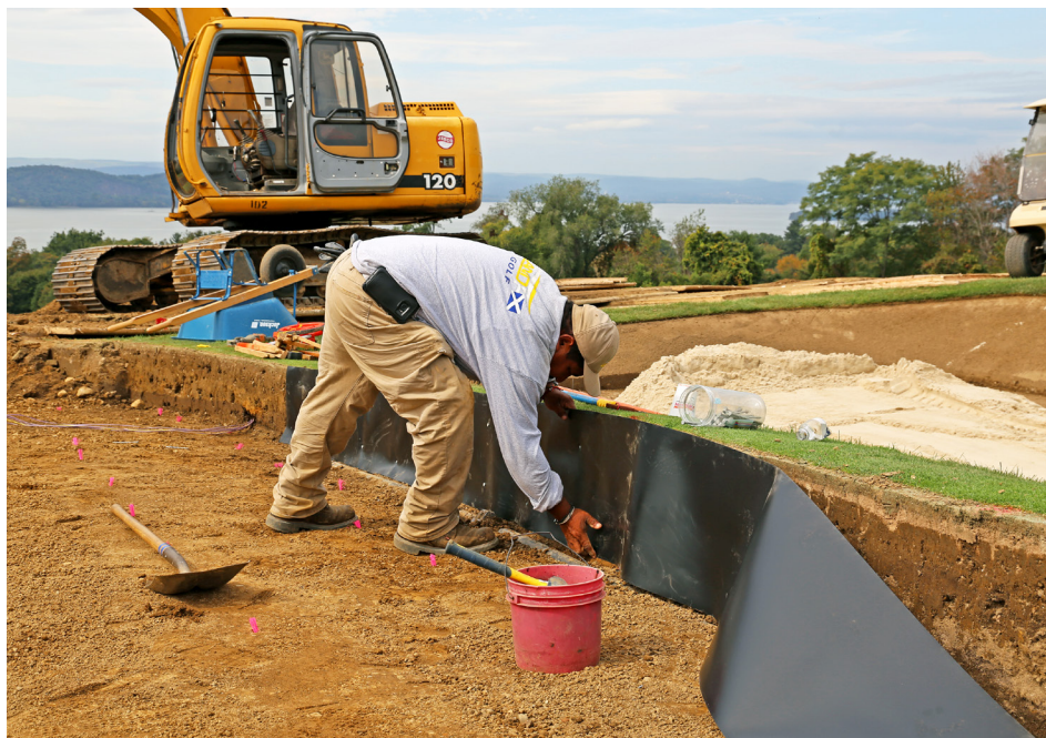
INSTALLING A WICKING BARRIER ALONG THE PUTTING GREEN CAVITY WALL IS OPTIONAL BUT MAY IMPROVE MOISTURE MANAGEMENT IN CERTAIN CIRCUMSTANCES.
