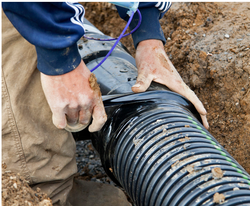
DRAINAGE PIPES SHOULD BE JOINED USING SPECIALIZED CONNECTION FITTINGS. MANY CONTRACTORS WILL SECURE EACH CONNECTION WITH TAPE TO PREVENT SEPARATION.
