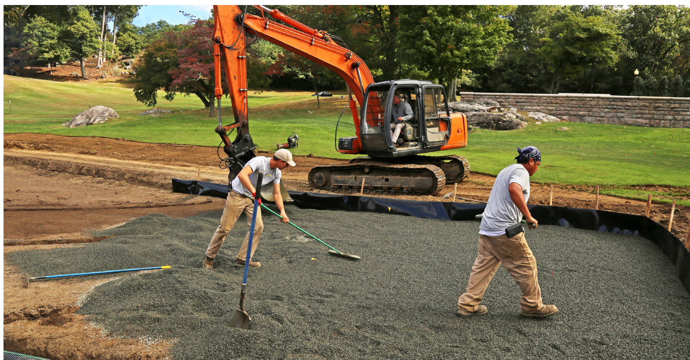
THE GRAVEL LAYER SHOULD BE SPREAD TO A MINIMUM DEPTH OF 4 INCHES. THE SURFACE OF THE GRAVEL LAYER SHOULD MIRROR THE FINISHED SURFACE OF THE PUTTING GREEN.
