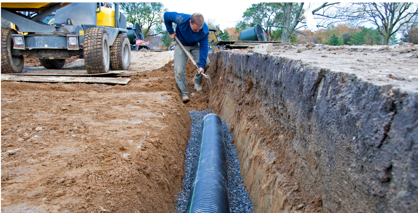
PERIMETER DRAINS – i.e., SMILE DRAINS – SHOULD BE INSTALLED IMMEDIATELY AGAINST THE CAVITY WALL.
