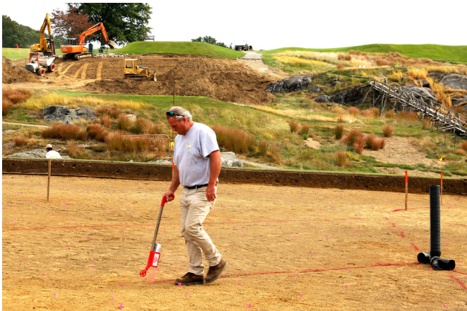
SPRAY PAINT AND A MARKING GUN MAKE IT EASY TO LAY OUT DRAINAGE LINES.
