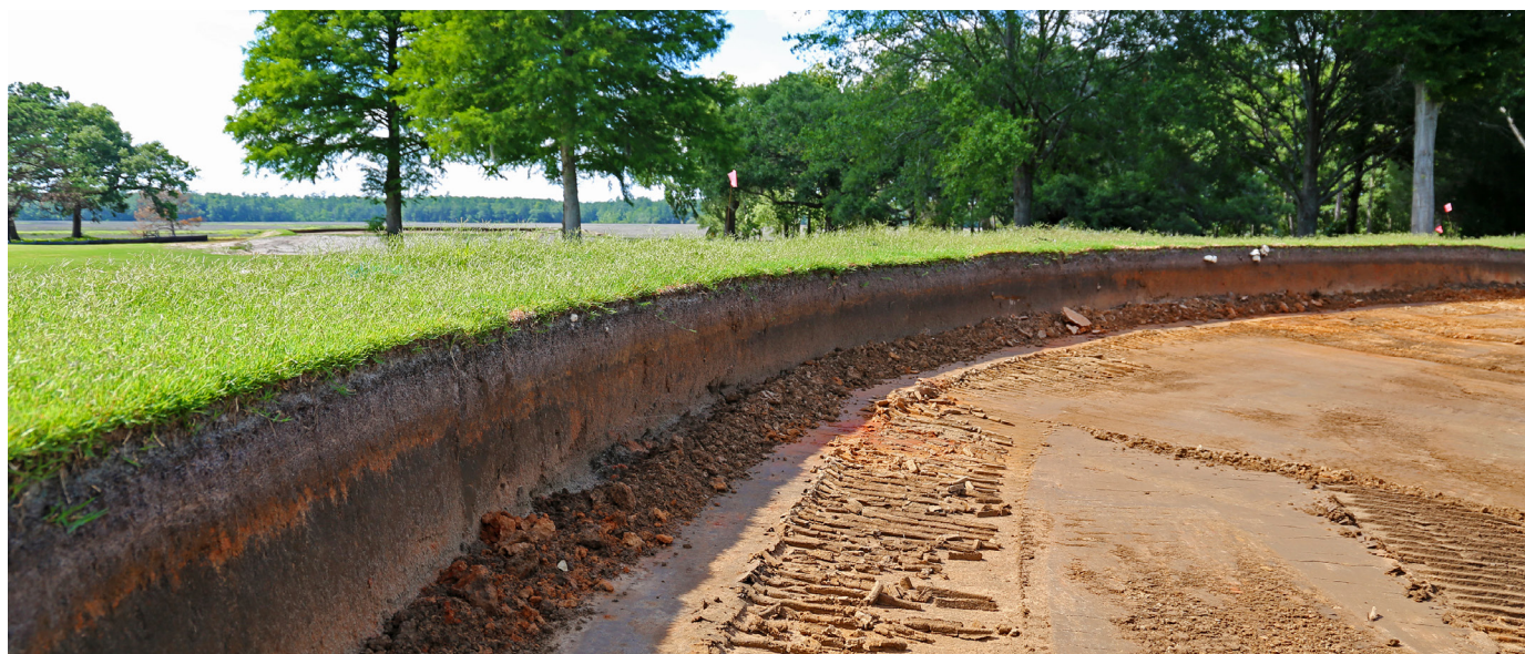
CAVITY WALLS SHOULD BE AS CLOSE TO 90 DEGREES TO THE CAVITY FLOOR AS POSSIBLE. COLLAR AREAS SHOULD ALSO BE INCLUDED WITHIN THE PUTTING GREEN CAVITY.
