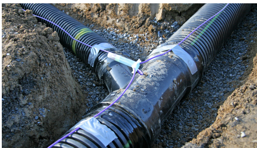
IF A LOCATOR WIRE IS INSTALLED IN EACH DRAINAGE TRENCH, A WIRE-TRACKING DEVICE CAN BE USED TO QUICKLY LOCATE THE DRAINAGE SYSTEM AFTER IT HAS BEEN BURIED.
