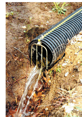
The end of drainage lines must be protected to prevent animals from entering the pipe.
