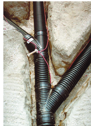
Lay a #14 irrigation wire in each ditch to allow easy location at a later date using a wire tracking device.
