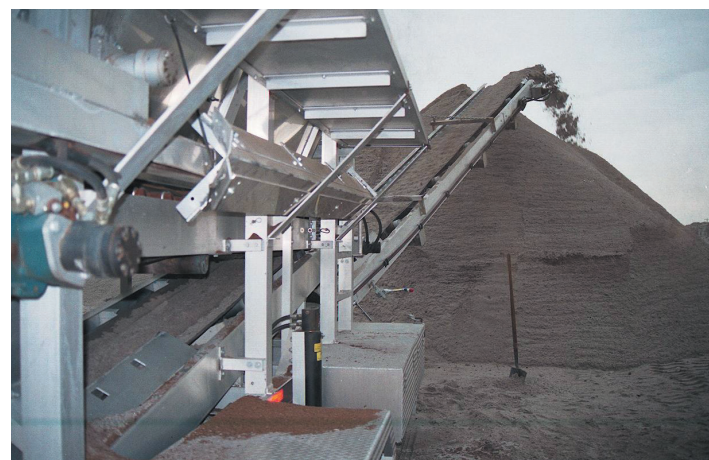
Blending the rootzone materials at the plant provides numerous advantages over blending on the construction site.
