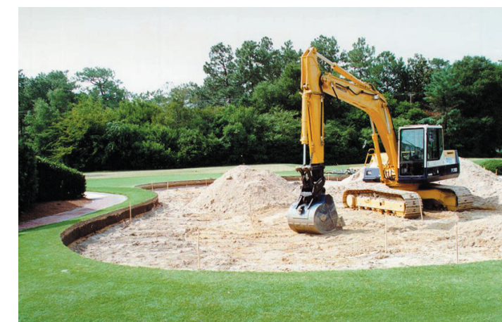
Shelling is a process that is frequently employed on existing greens when the previous contours of the green are to be preserved. In most cases, little work is done to the surrounding areas.
