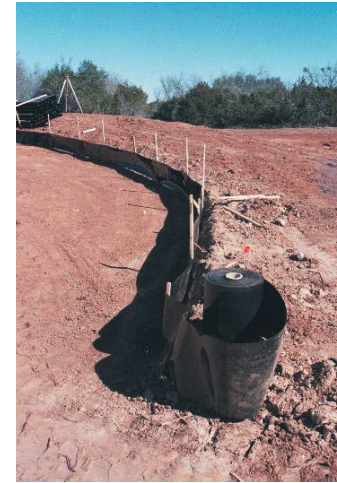
30 ml plastic can be purchased that makes the installation easier due to the stiffness of the material.
