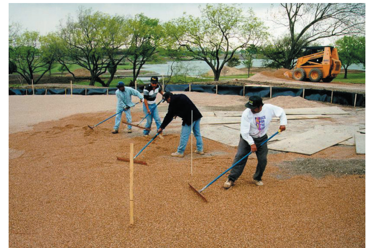
The gravel should be spread to a minimum depth of four inches and according to the grade stakes. The surface of the gravel layer should "mirror" the finished surface of the putting green.
