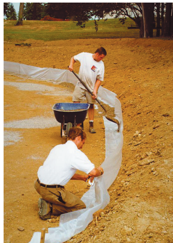
Gravel is added to the inside of the cavity over the plastic to keep it in place.
