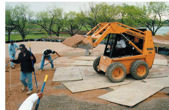
Heavy plywood is used to prevent damage to drainage lines from heavy equipment.
