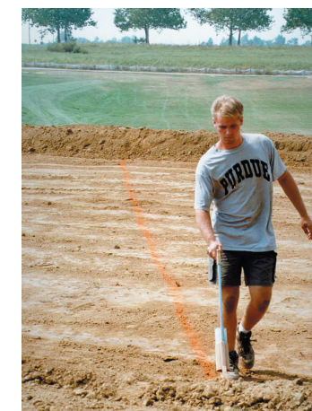
Spray paint and a marking gun make it easy to lay out the drainage line pattern.
