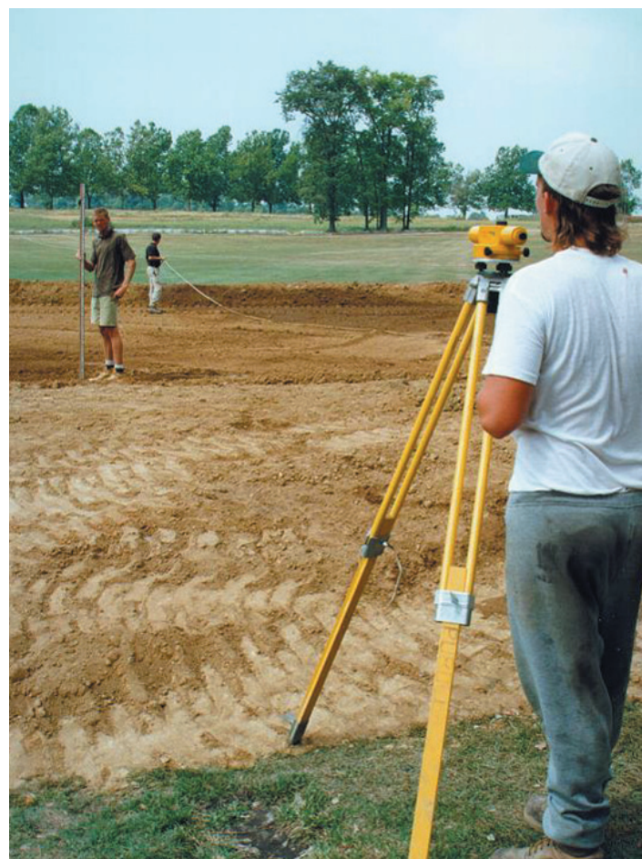
Use a surveying instrument to ensure the drainage ditches have at least 0.5% slope to the exit points.
