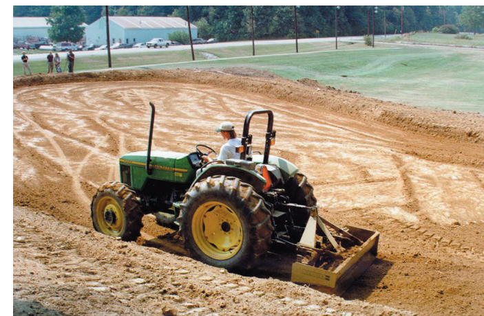
The extra time spent preparing the subgrade will result in a smooth, well-compacted base on which to build the remainder of the green.
