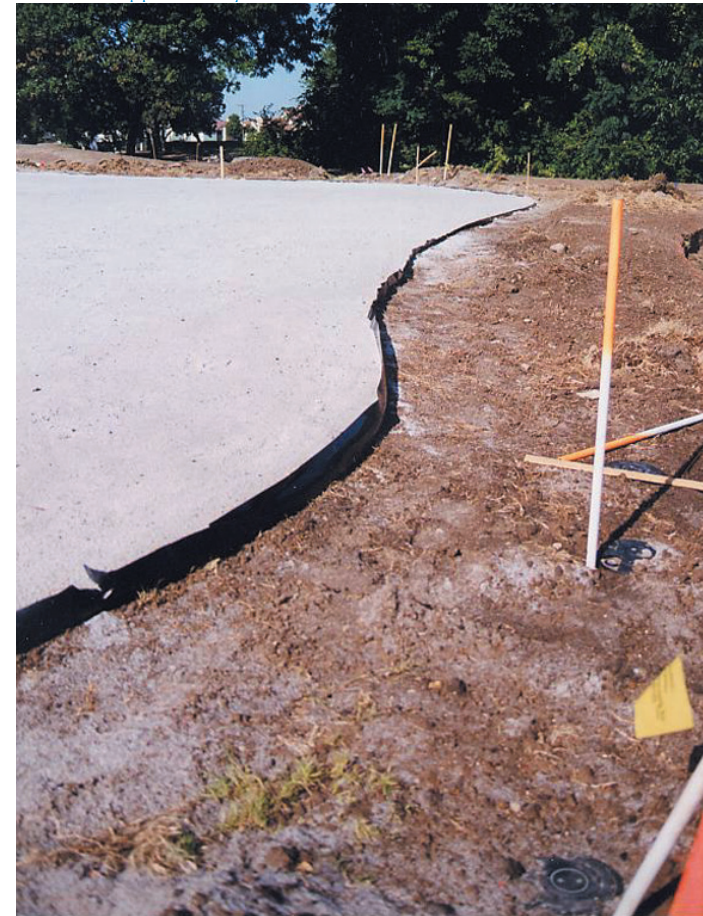
surrounding grade to help prevent soil from the surrounds from washing onto the green. It is removed later with a carpet knife or similar tool.
