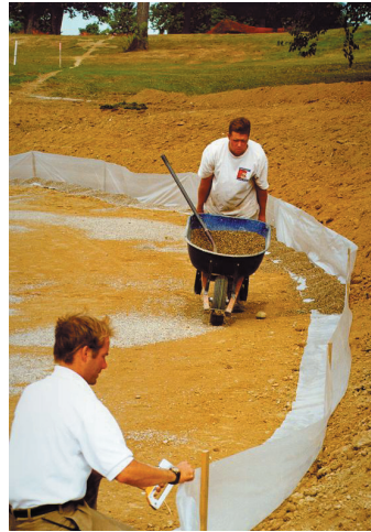
6 to 8 ml plastic sheeting is readily available from hardware stores and works fine for the wicking barrier.
