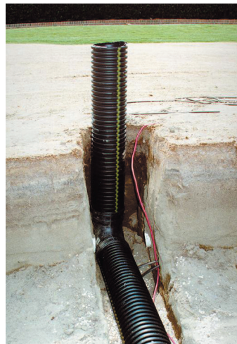
Exit the wire near the "clean-out" or near a sprinkler so the end of the wire can be found easily.
