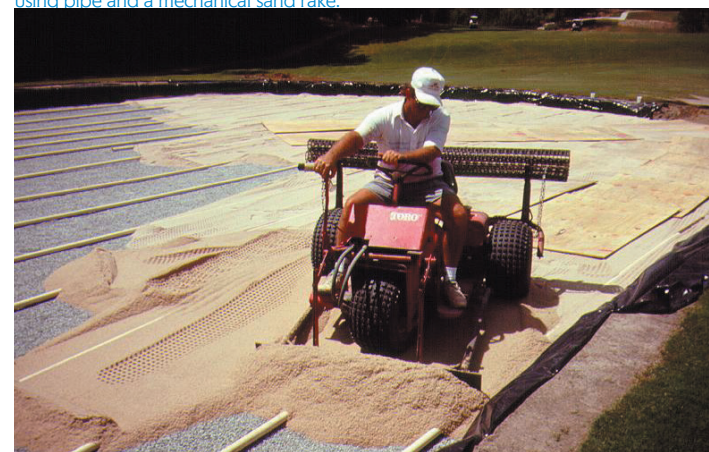
Tip 1: Locate gravel that is compatible with the rootzone mixture so that the intermediate layer can be eliminated — it
