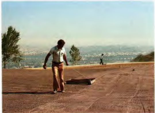
"Floating Greens" provides a smooth finished grade. A light golf cart can mechanize this job.
