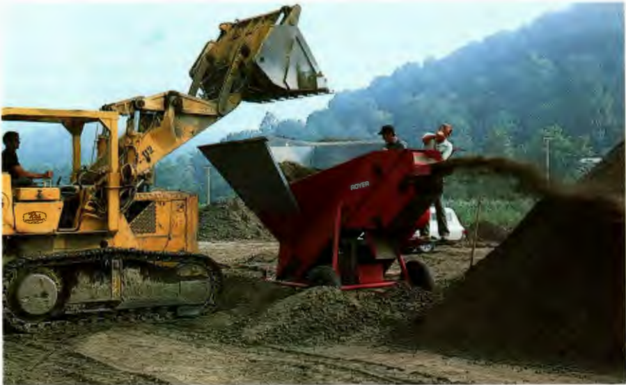
Off-site mixing is an essential feature of top mix preparation. The use of a shredder/mixer is one method available for ensuring a thorough blending of the top mix components.
