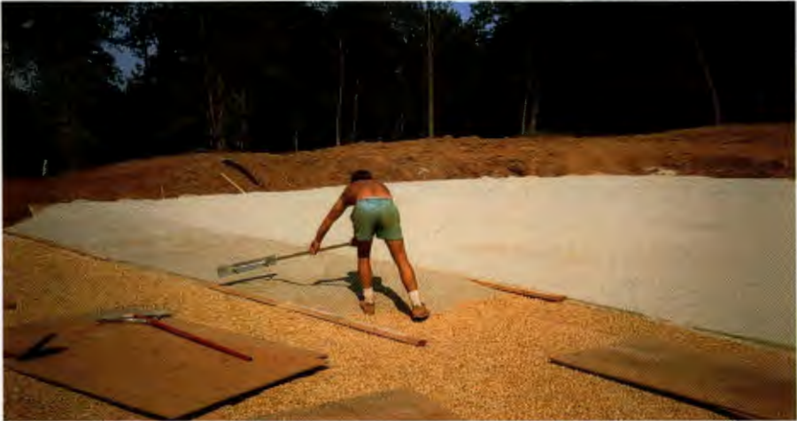
The two inch intermediate sand layer is easily spread by hand.
