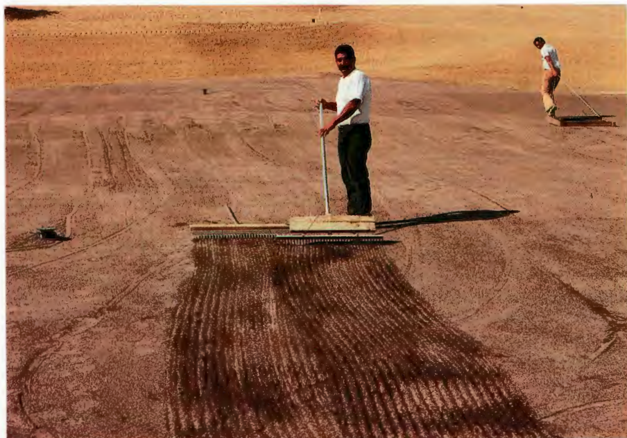
A light, continuous raking prepares an excellent, soft, seed bed.
