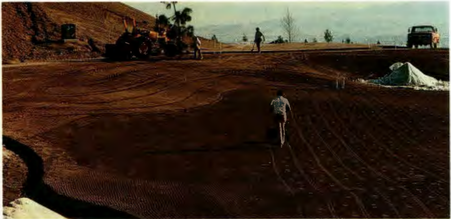
Seeding should be done at half rate in two directions to ensure uniform coverage.
