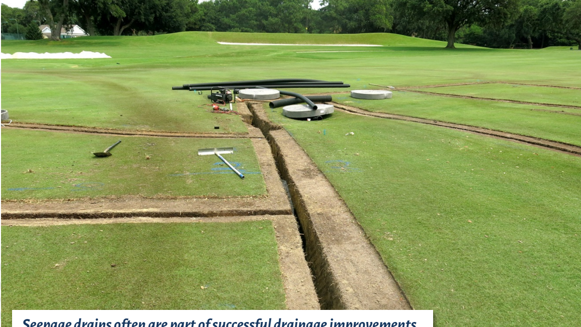
Seepage drains often are part of successful drainage improvements.
