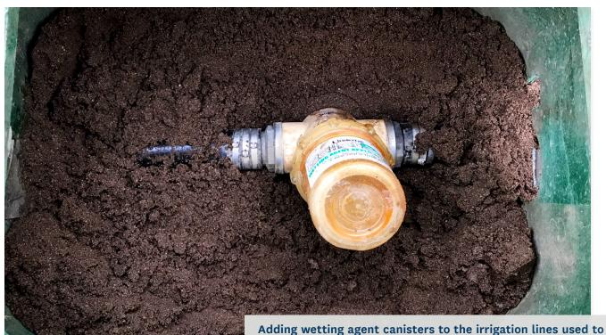
Adding wetting agent canisters to the irrigation lines used to water bunker banks has improved turf conditions and saved staff time at Point Judith.
